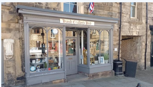
Timber shopfront with stone base to stallriser
